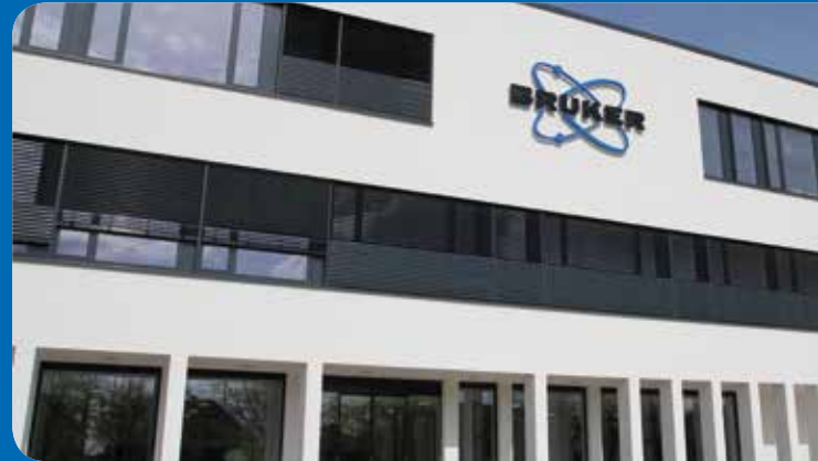
Bruker facility in Karlsruhe
